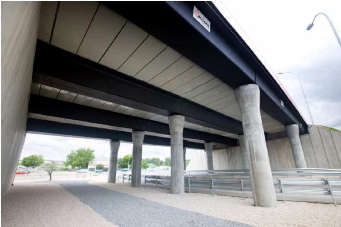
Figure 116 Overview of M 111 Bridge (Burgos Muniz 2012)
