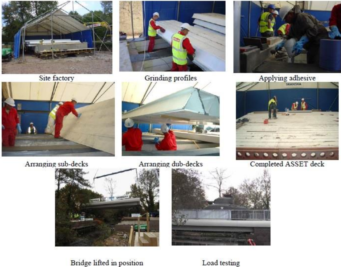
Figure 112 Manufacture process of the deck (Täljsten 2007)
