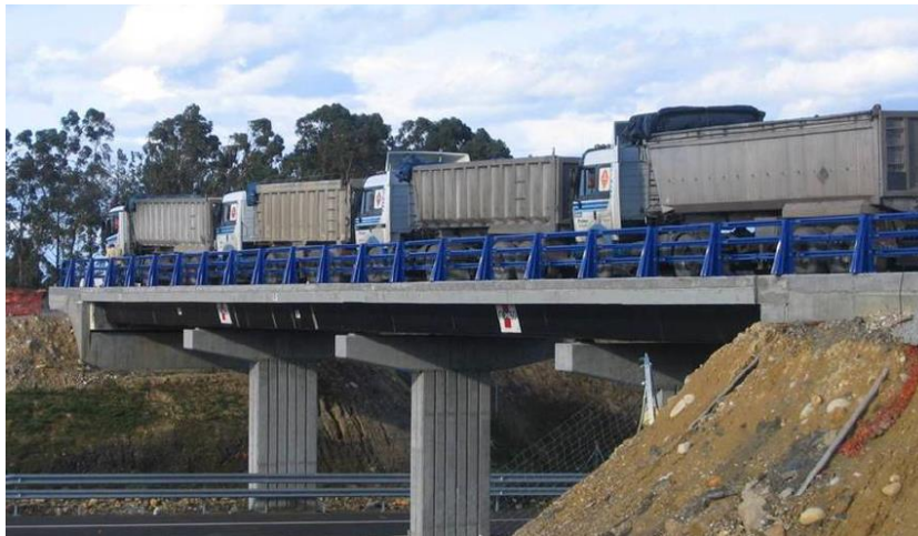
Figure 101 Heavy trucks placed on the PUMACOM Bridge - the static load test (Muniz & Bansal 2009)
