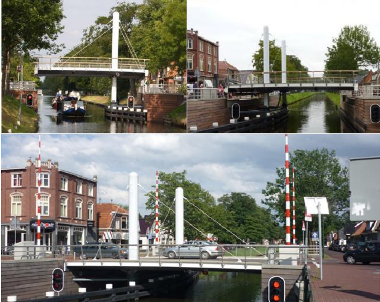
Figure 125 Overview of the Oosterwolde heavy traffic lift bridge (Fibre core Europe 2010; Chlosta 2012)
