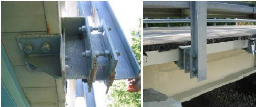
Figure 171 Guardrail with steel connection (Hastak et.al 2004)
