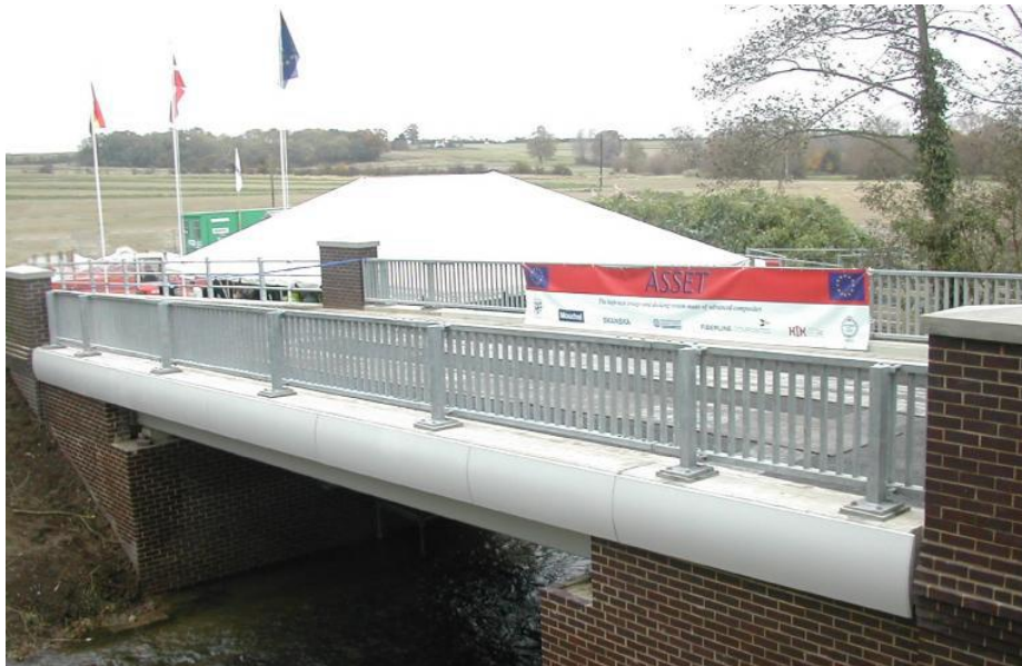
Figure 108 Overview of West Mill Bridge (Canning 2012)
