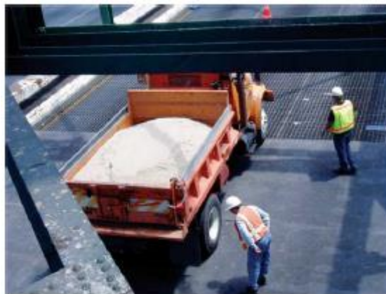
Figure 87 Visual inspection with dump truck placed on deck (Meyer 2006)
