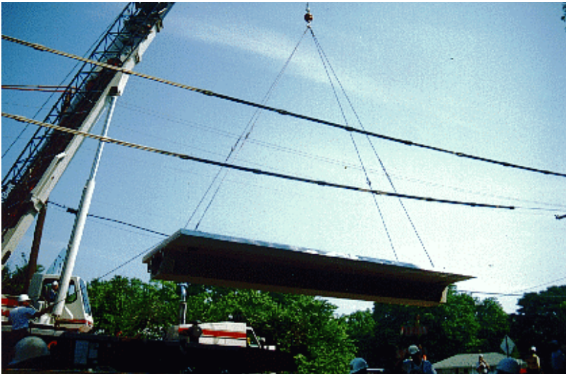
Figure 106 Beam element hoisted in place by crane (BCEO 1998)
