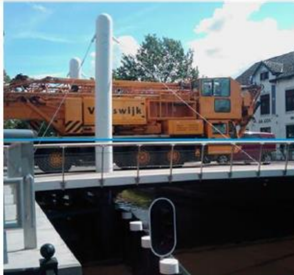
Figure 126 The lift bridge withstands load from heavy trucks (Fibre core Europe 2010)
