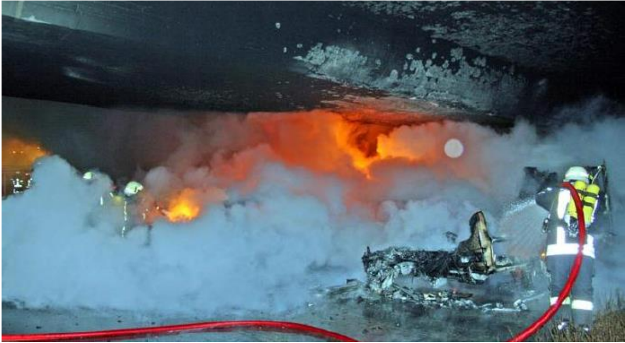
Figure 41 A bridge fire in Germany (Chlosta 2012, p. 135)
