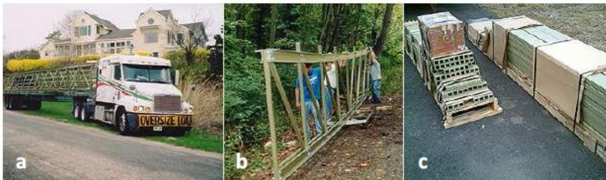
Figure 80 Pultruded profiles as a) fully assembled b) partially assembled c) separate components (Potyrala 2011, p. 27)
