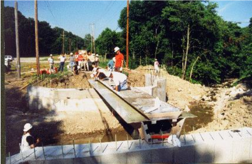
Figure 105 Installation of the middle beam (BCEO 1998)
