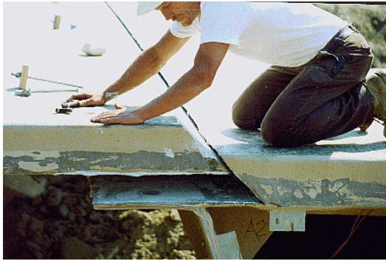
Figure 107 Constructor sets the bridge in place (BCEO 1998)
