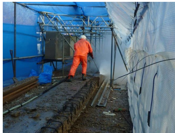
Figure 2 High pressure water blasting (source: APA concrete repairs Ltd.)
