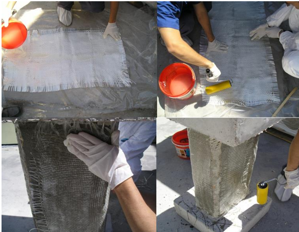
Figure 14 Wet layup process (Mostostal Warszawa S.A.)
