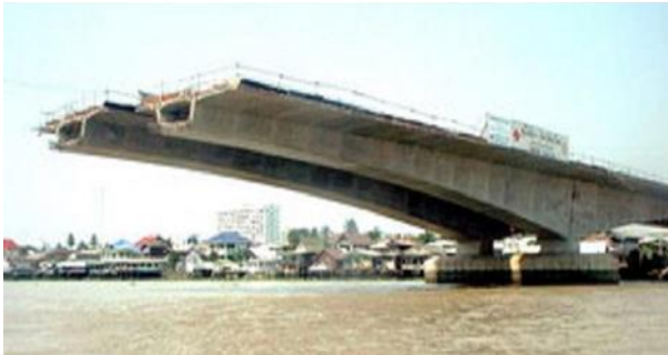
Figure 28 Top left: post-tensioned concrete bridge constructed with incremental launching [6]; Bottom left: post-tensioned concrete bridge erected with cantilever method [6]; Right: cable in aluminum ducts in the formwork (photo by Störfix)
