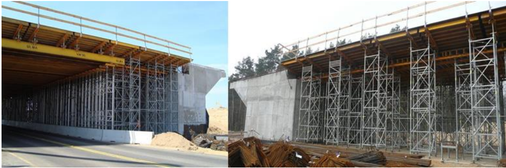
Figure 29 On-site fabrication of reinforced concrete bridges
