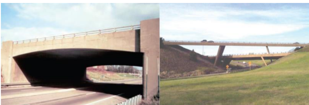
Figure 42 Examples of the single and multi-span concrete frame bridges. On the left frame shape type “U” and on the right K-frame
