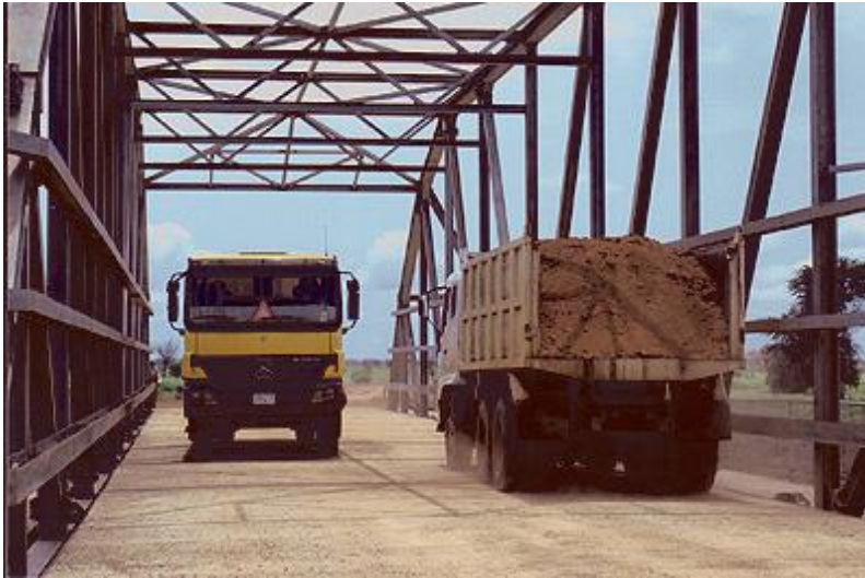
Figure 10 Through truss bridge (name and place of the bridge are unknown) [1].
