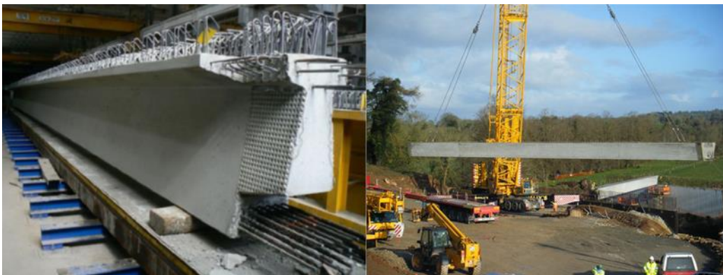
Figure 27 Pre-tensioned concrete beams and their installation on the building site
