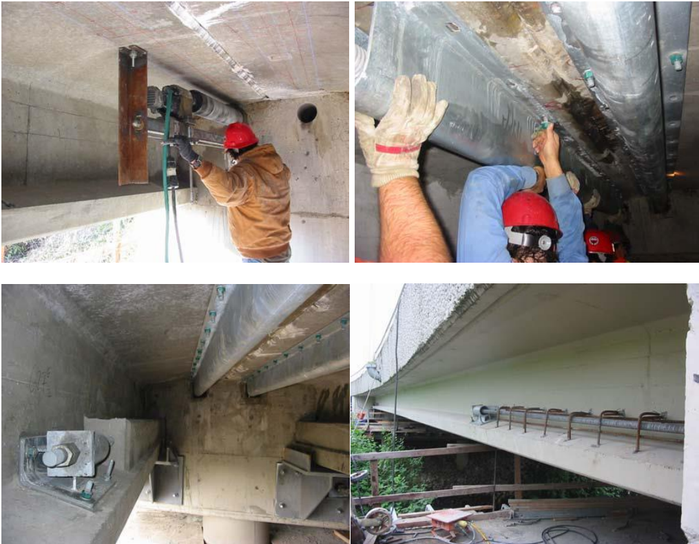
Figure 8 External post-tensioning [1]
