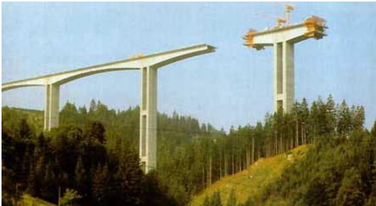
Figure 37 Concrete box beam bridge erected with balanced cantilever method
