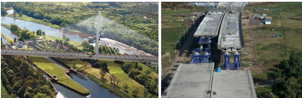
Figure 43 Reinforced concrete cable-stayed bridge in Wroclaw in Poland constructed by Mostostal Warszawa S.A in 2011
