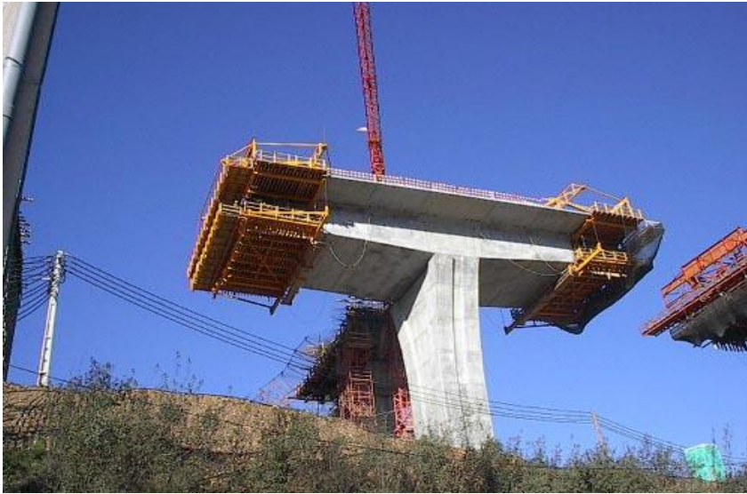
Figure 44 Erection of concrete cable-stayed bridge with cantilevering method
