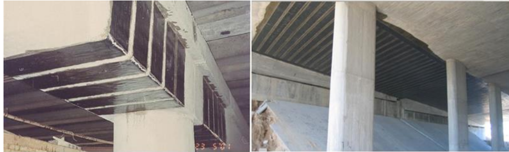
Figure 16 Reinforced bridge using S&P carbon tapes
