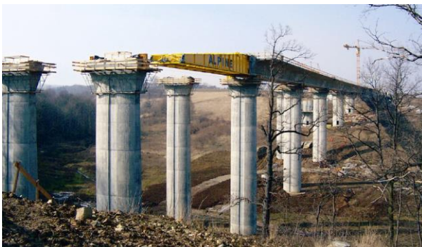
Figure 38 Concrete box beam bridge during construction with incremental launching
