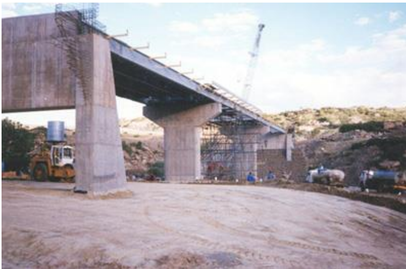
Figure 3 Erection of continuous steel beam bridge [1]
