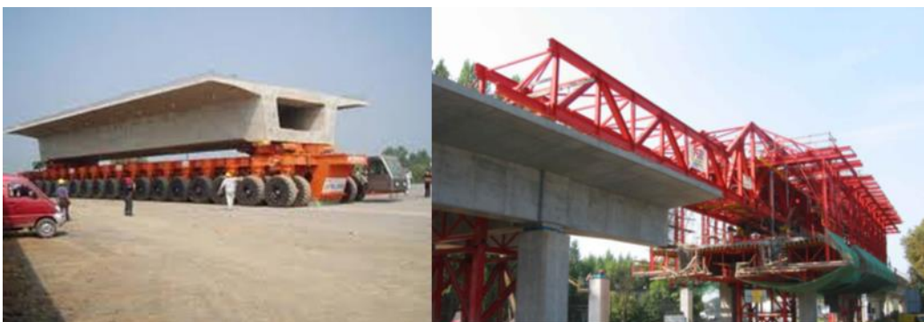
Figure 36 Left) precast box-beam, Right) traveling gantry [4]
