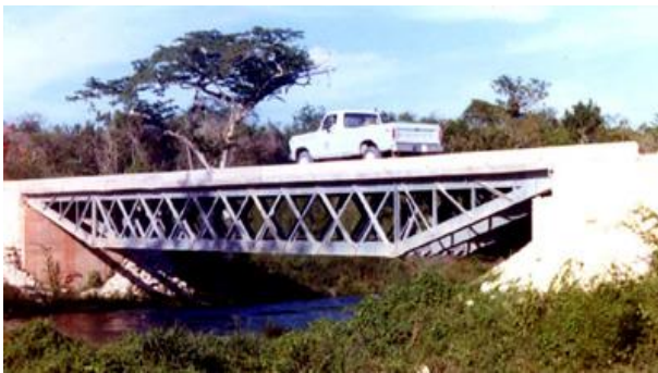
Figure 5 An example of steel over truss bridge [1]
