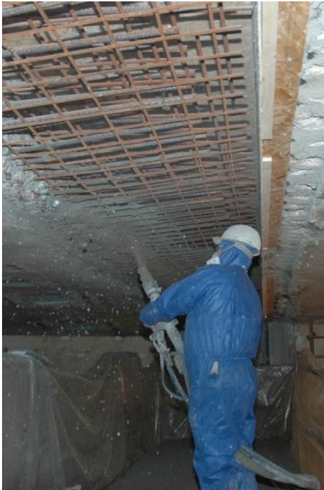
Figure 3 Shotcrete (wet) (source: VTG Beton)
