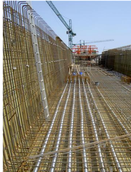
Figure 28 Top left: post-tensioned concrete bridge constructed with incremental launching [6]; Bottom left: post-tensioned concrete bridge erected with cantilever method [6]; Right: cable in aluminum ducts in the formwork (photo by Störfix)
